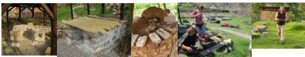
Building of traditional oven
